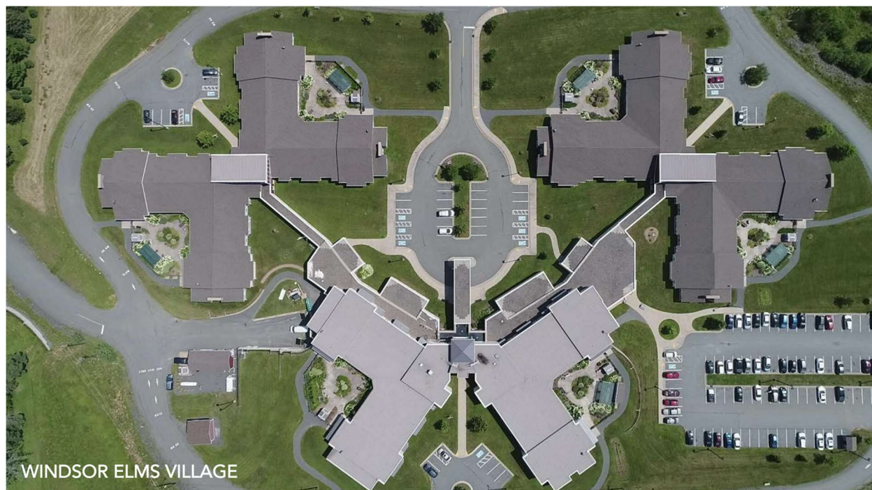
Figure 7: Windsor Elm Village Aerial Photo. Source: Equilibrium Engineering (n.d)
