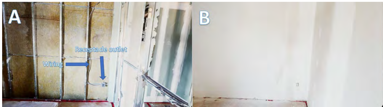
Figure 14 Side-by side comparison of meshes taken from within the VR app, making an example of its use to find electrical component routing behind drywall. Scan 1 is in frame A, and Scan 3 in frame B.
